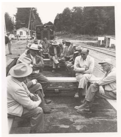
Railroad being built
